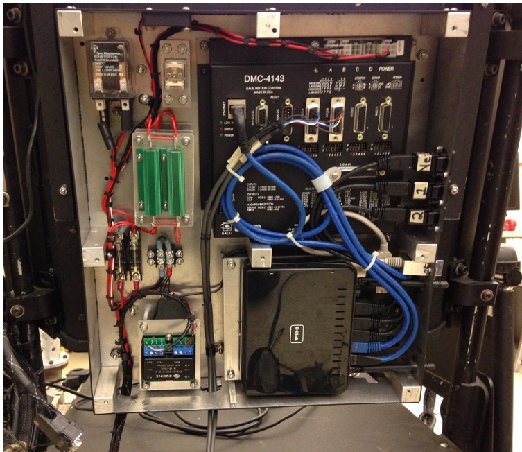
Galil Motion Control DMC41x3 Board installed in wheelchair control box
